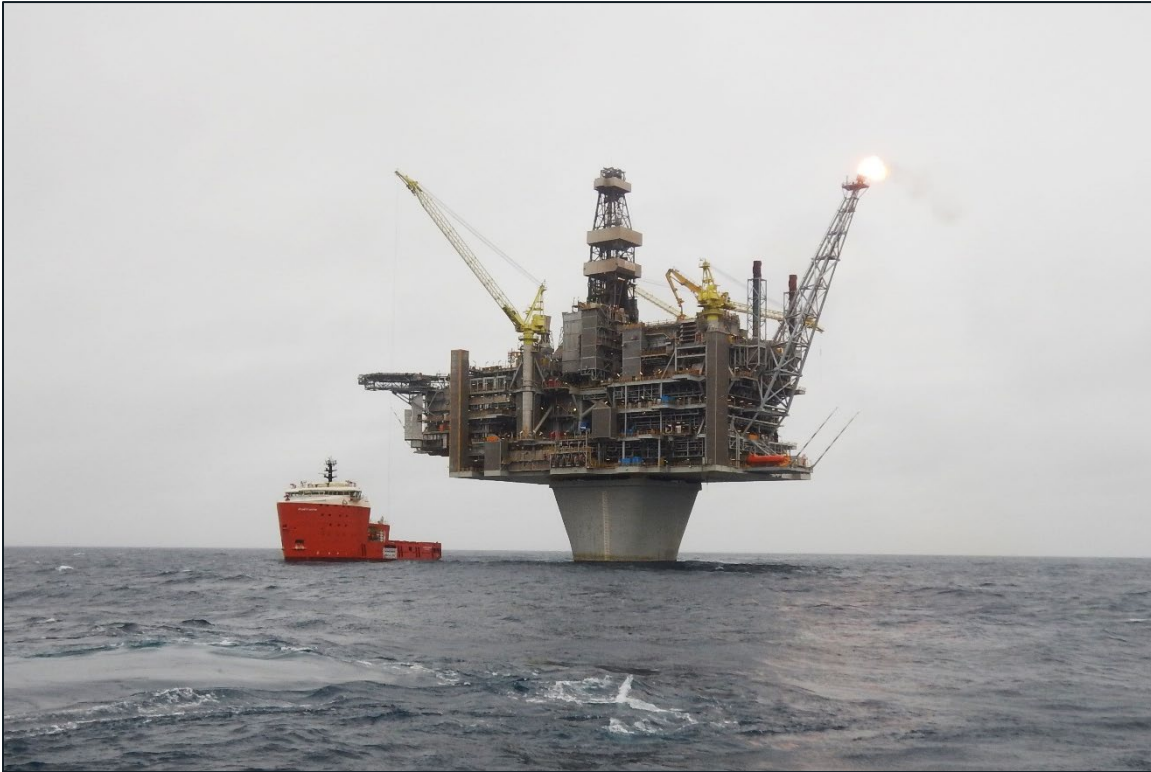
Figure 1-2 Hebron Platform in August 2019 with the MV Atlantic Griffon offshore supply vessel on the left.
