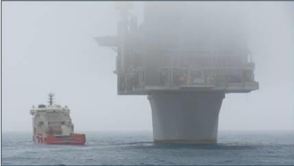
Figure 1-2 Hebron Platform with the OSV Atlantic Griffon offshore supply vessel on the left.
