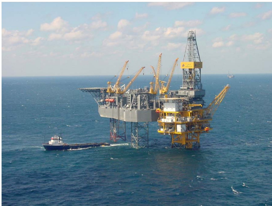
Figure 3.5 Rowan Gorilla VI operating with 673' leg length over production platform.
